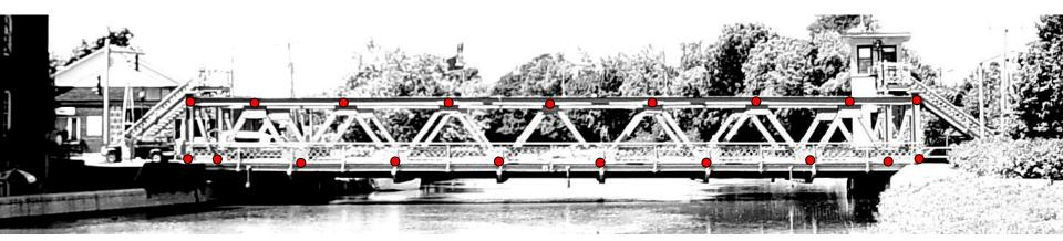
Each side of the main street bridge in Brockport, NY has 19 joints, 35 members, and three reaction forces (pin and roller), making it a statically determinate truss.
